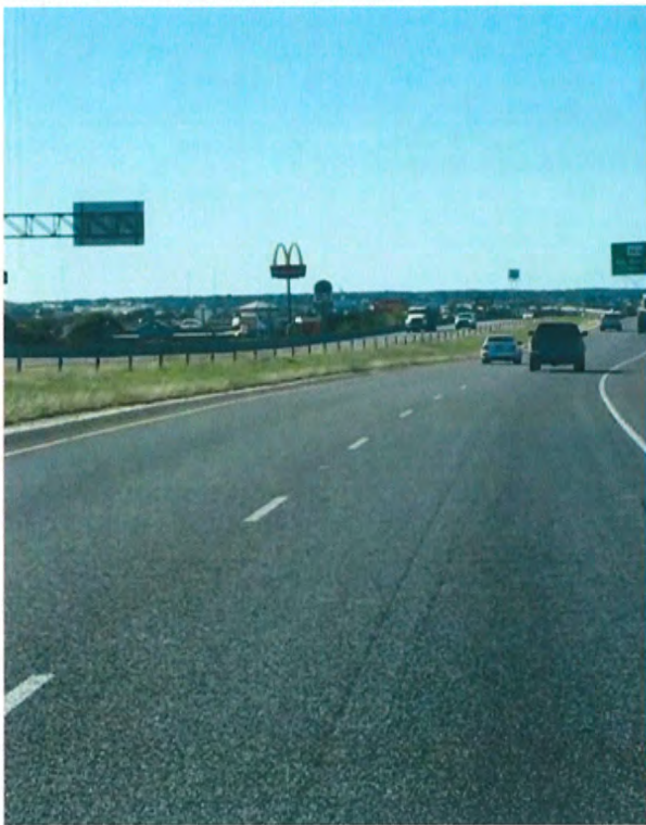
Westbound 71, South side of 71
